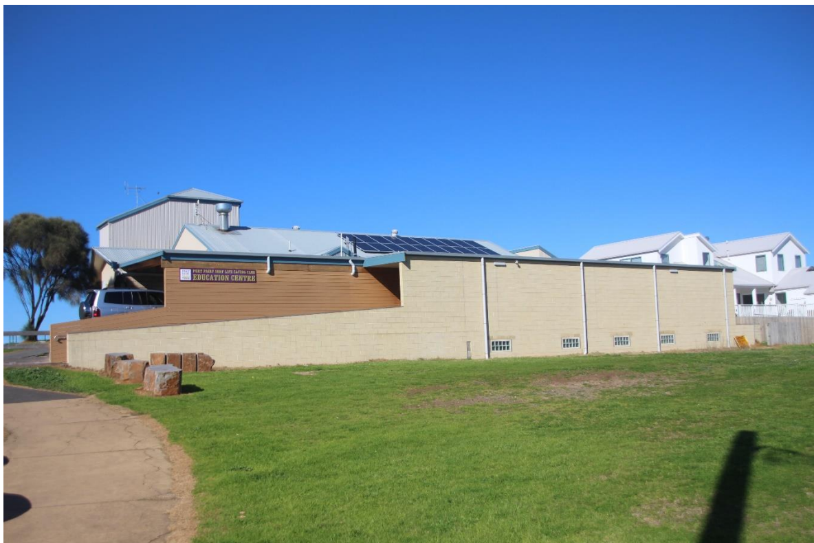
Entrance to the new Education Centre from Hughes Avenue
