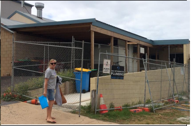
Ramp entrance with Martina checking out progress
